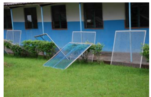
Repairing mosquito screens
