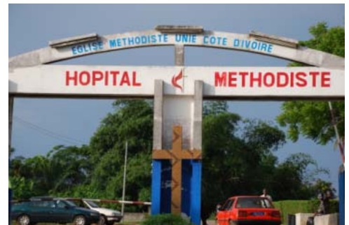
Main entrance to Hospital
